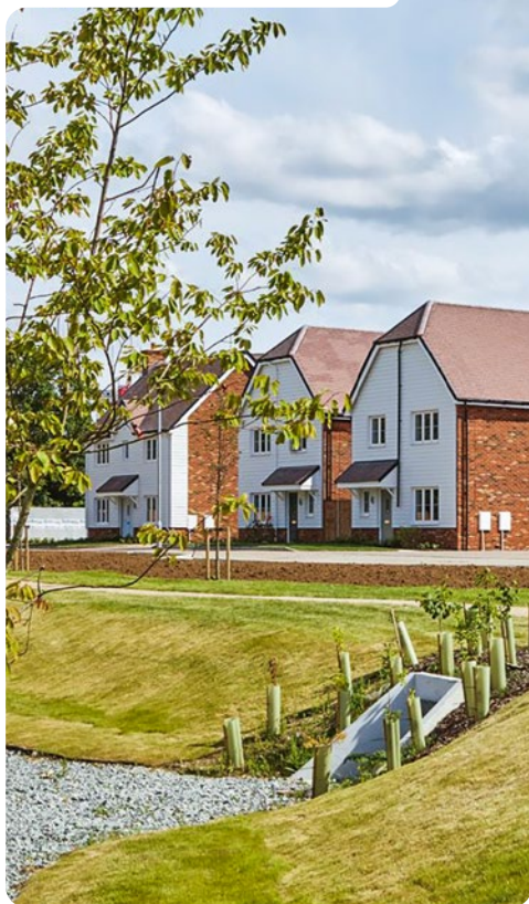
Street scene of Highlands Grange, Swanley.
